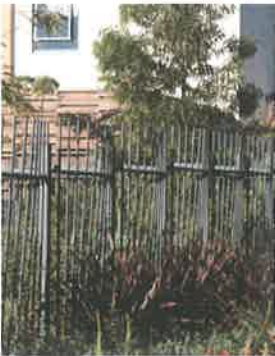
PALISADE STEEL FENCES
